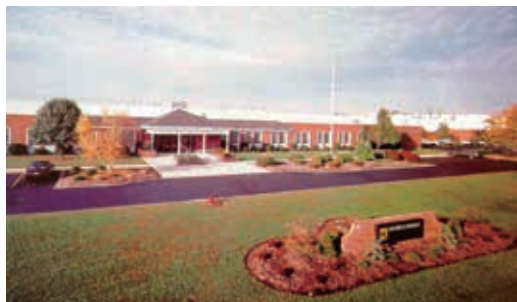
Square D facility in Oxford, Ohio U.S.A. is an ISO 9001 and ISO 14001 registered busbar trunking manufacturing facility.
